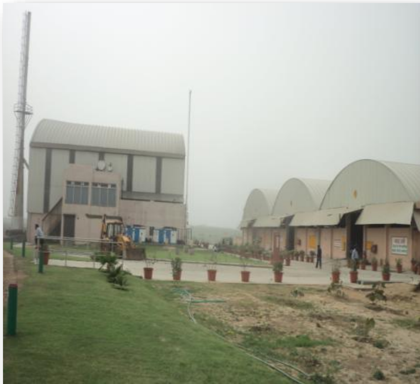
Overview of Facility -Haryana
