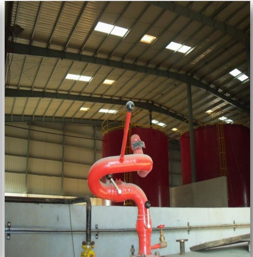
Fire Hydrant System
