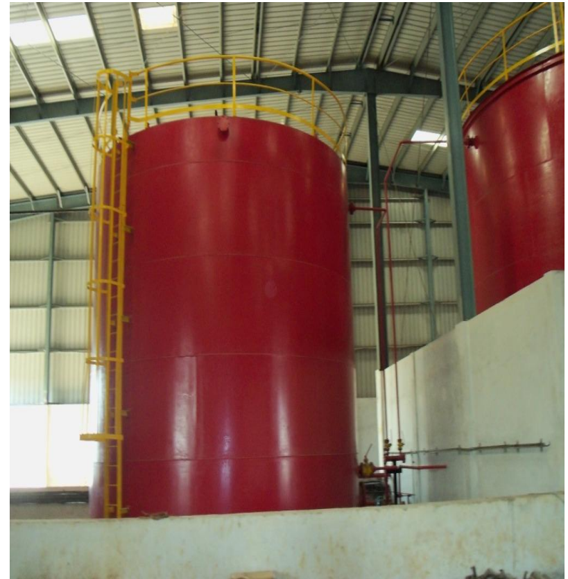
Liquid Storage Facility
